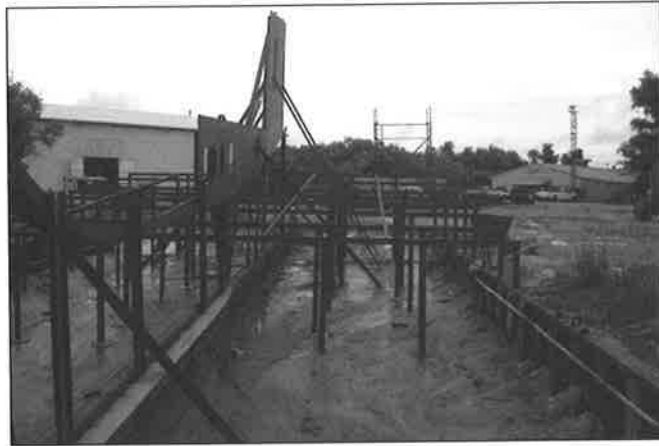
Figure 11: First Z-Tech 7500 commencing construction at Main Iron Works.
