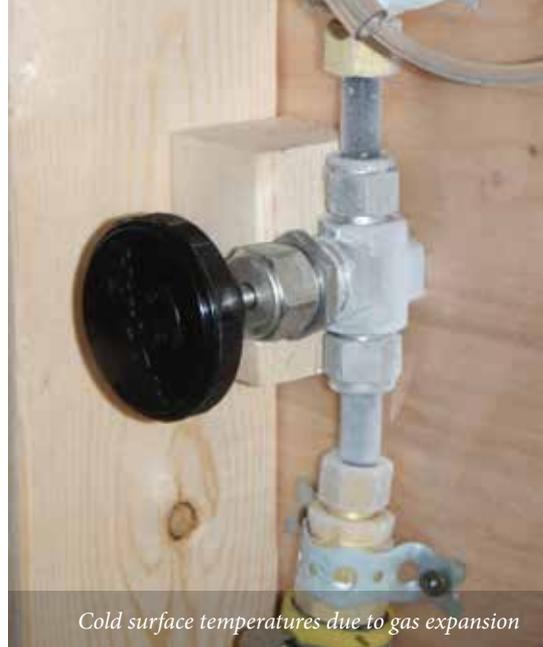
Cold surface temperatures due to gas expansion
